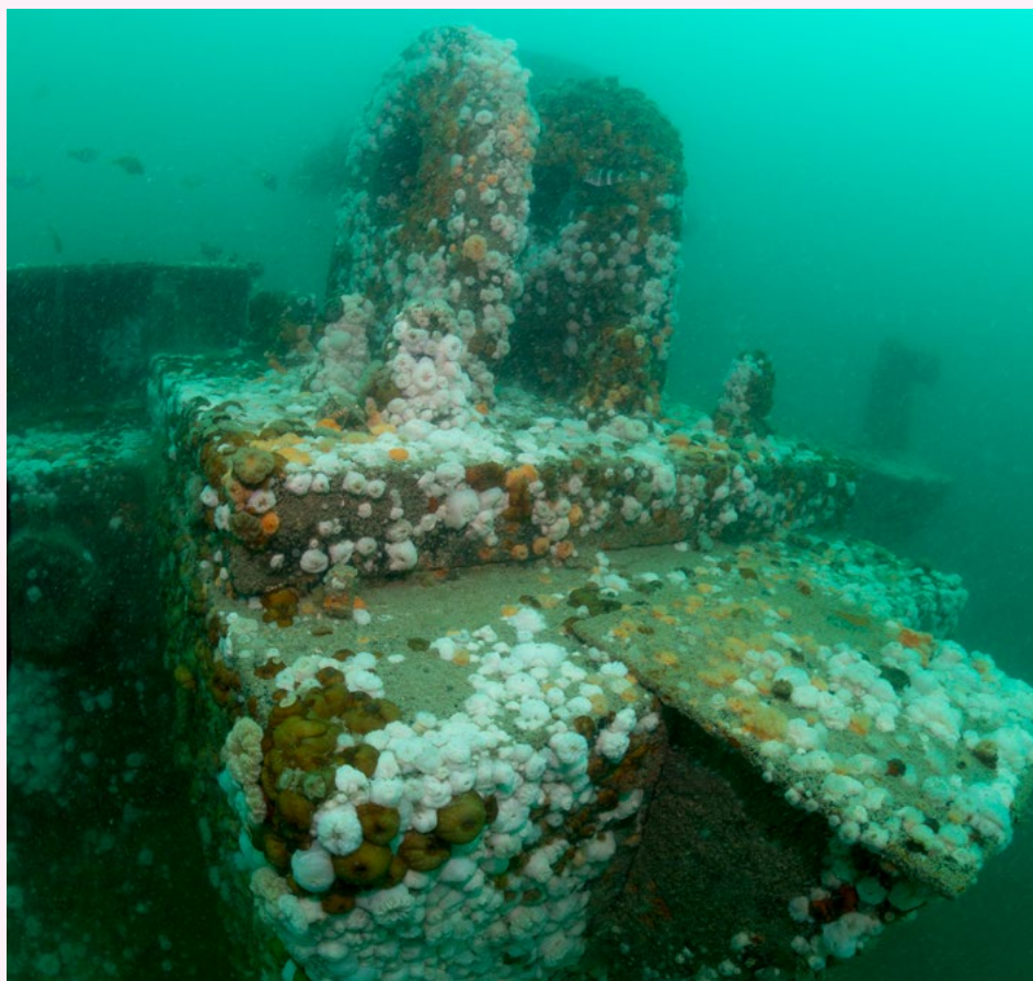
Part of the overgrown base of the disused Halfweg gas platform. Photo Udo van Dongen, Bureau Waardenburg
