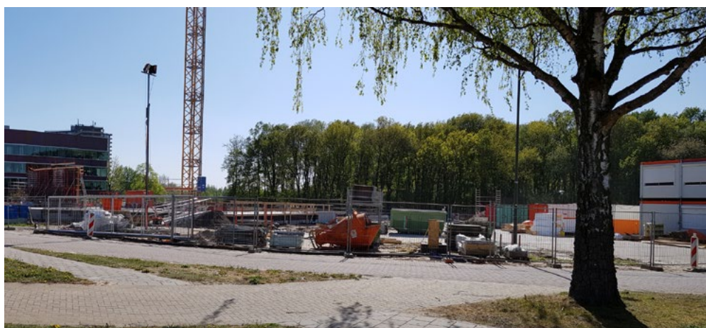
▲ The third education building under construction.
