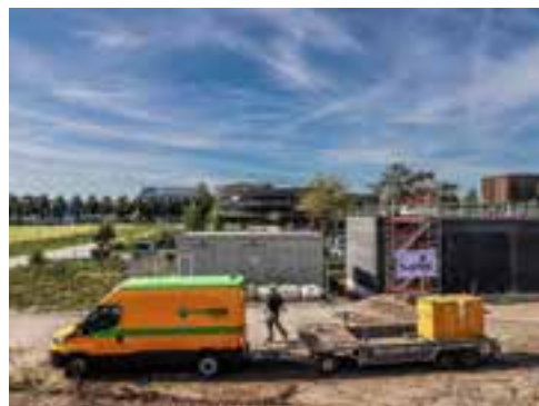
▲ The new transformer station under construction.
