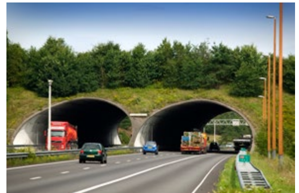
▲ The wildlife crossing over the A50 motorway at Woeste Hoeve.
